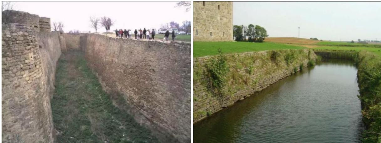
Fig. 3. Dry ditch and a ditch filled with water.
